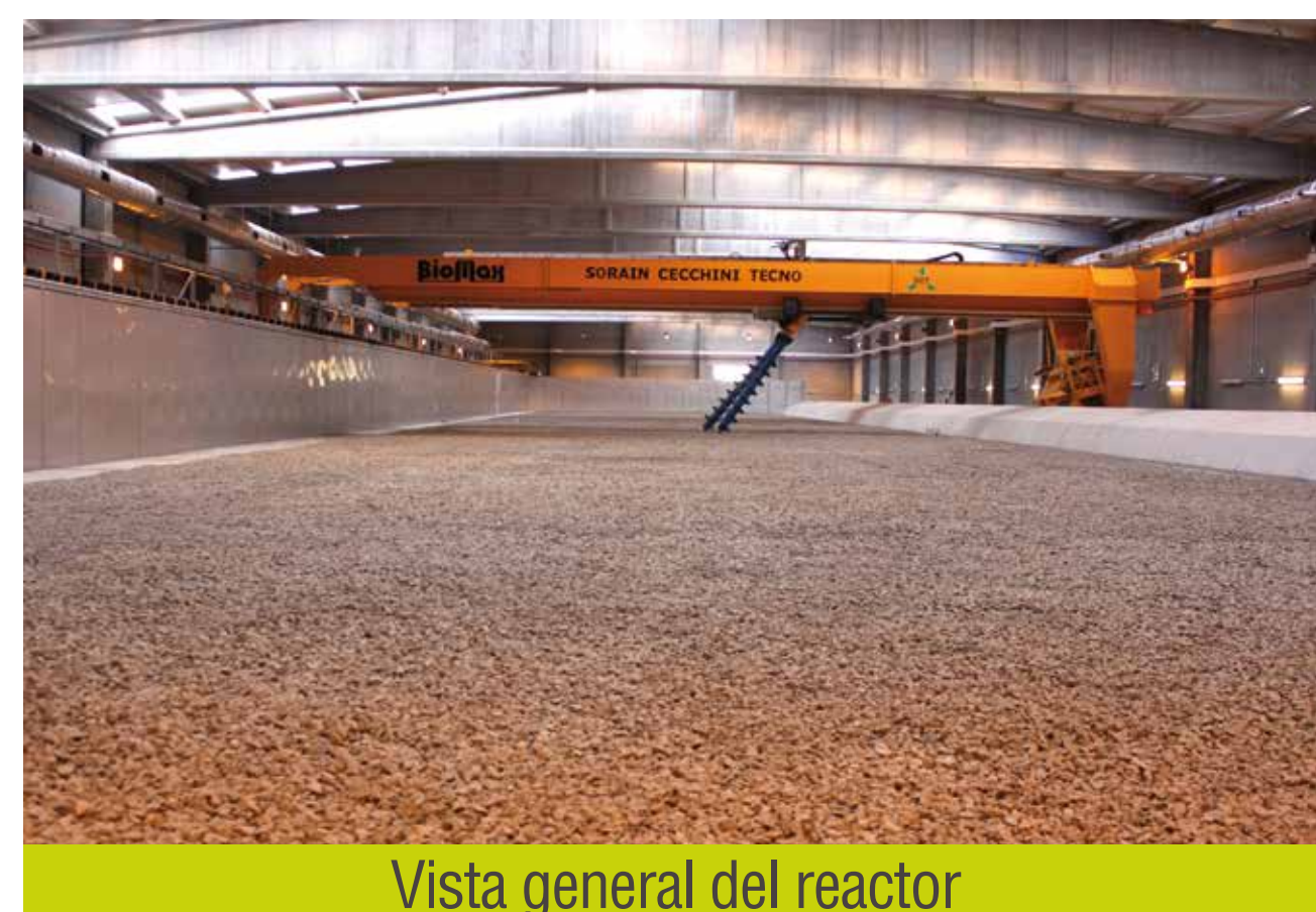
Vista general del reactor
